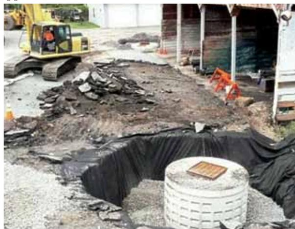
Pavement is removed and the first dry well is installed.
