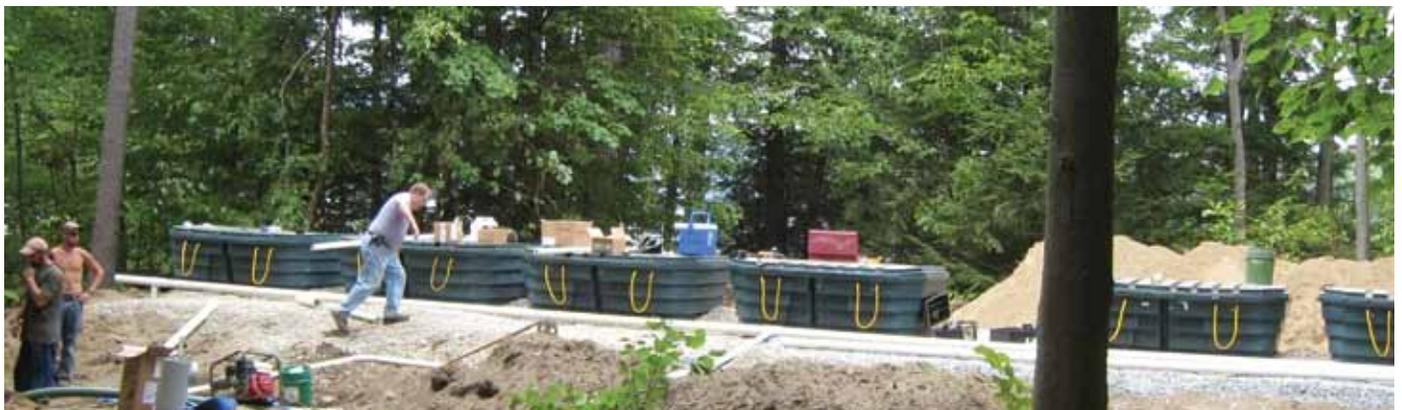
Seven peat containers are readied for level installation on Oahu Island. Above, the completed project (you can just see the top of the units on the crest of the mound.)
