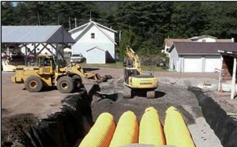
Infiltration chambers are in place and getting backfilled with stone. A double stacked dry well is in the upper right corner.
